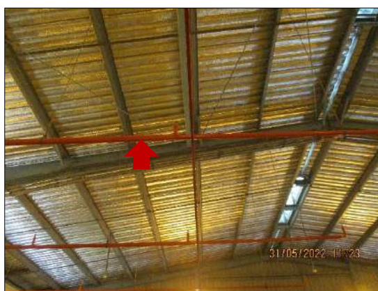
Water Deluge System / Water Spray System
